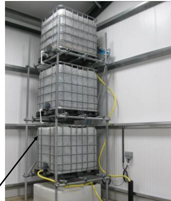
Biofilter within sprayer store / fill area
