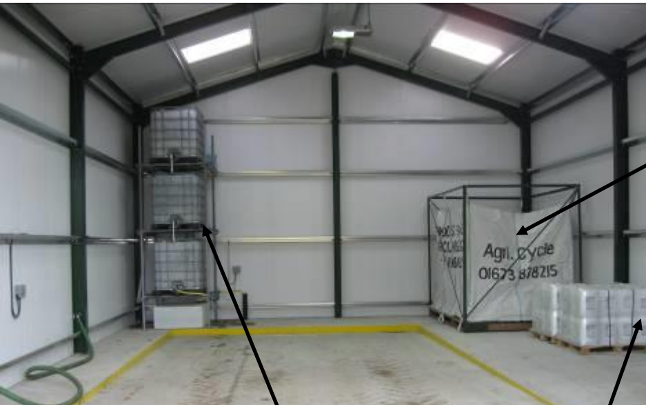
Fill area bunded below access level, building includes and biofilter & chemical store
