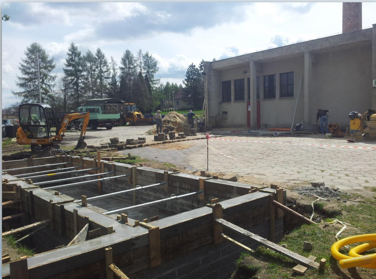
Concrete neutralizer chamber under construction.
